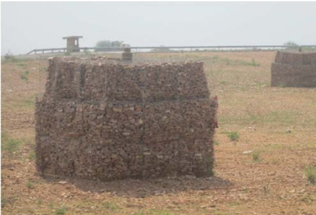
Figure 4. Gas extracting structure at Kpone landfill © 2013.
