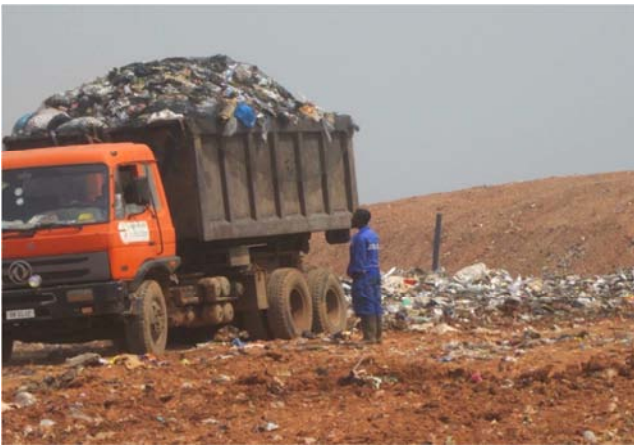
Figure 2. A spotter at the working face of Kpone landfill directing unloading trucks © 2013.
